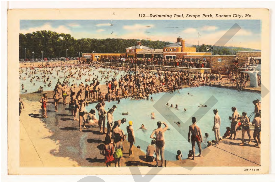
Figure 15. Circa 1941 postcard showing the Swope Park Swimming Pool at 6700 Lewis Road (extant), view southeast. Source: Kansas City Public Library Missouri Valley Special Collections.
