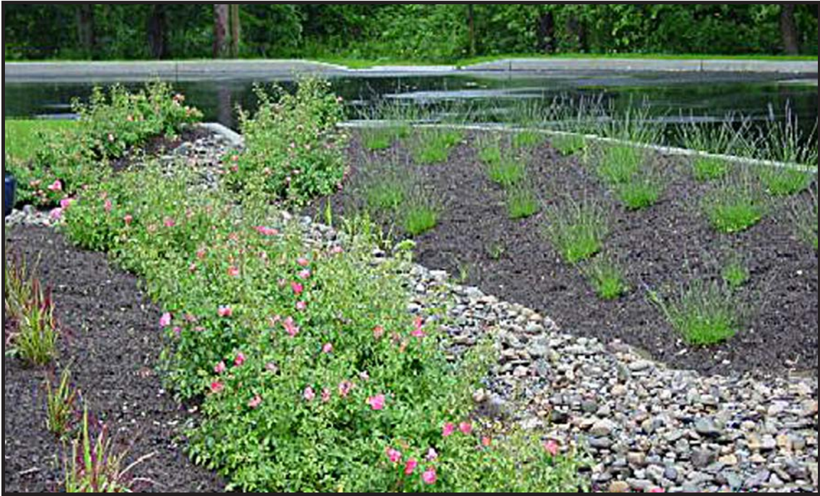
Figure 6.3 Biofiltration infiltration trench, Cumberland County, PA. Source: Pennsylvania Department of Environmental Protection
