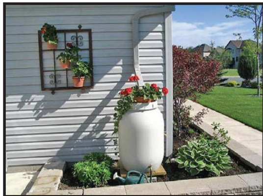
Figure 2.14: Residential rain barrel. Source: ABCs of BMPs
