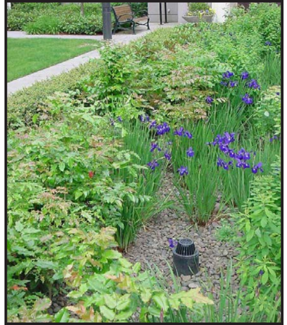
Figure 6.2 Infiltration Basin. Source: David Dods
