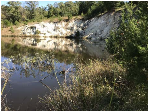
Reclaimed clay pit with a consolidated highwall as part of a wildlife post-mining land use.
