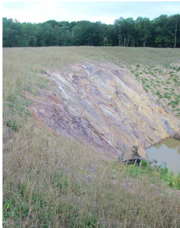
Reclaimed slopes surrounding a consolidated highwall.
