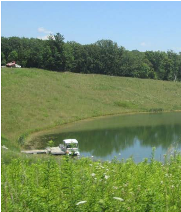
Reclaimed clay pit with stable slopes surrounding a water impoundment.
