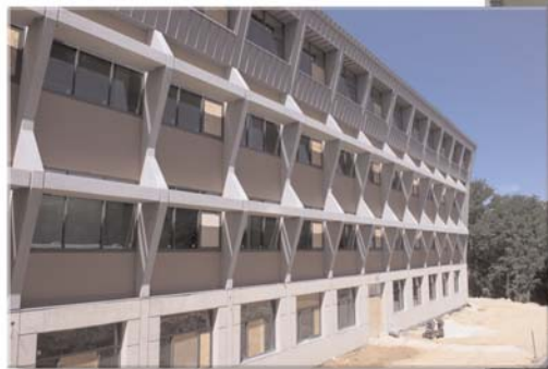
Building front as it appeared during construction in summer, 2004. Interior view of the front windows shows light shelves and sun shades already at work.
