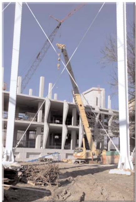
Facility support beams near completion in the fall of 2003.
