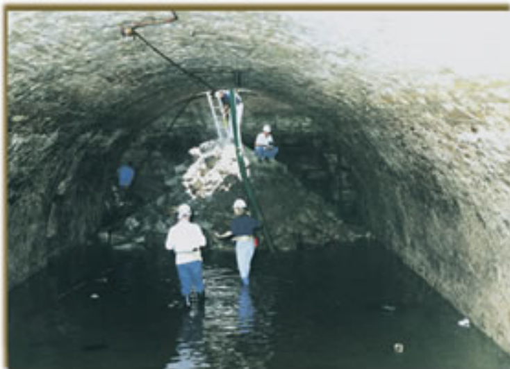
Sinkholes can be caused by man-made structures, such as this abandoned wine cellar in St. Louis. DNR photo by Jim Vandike
