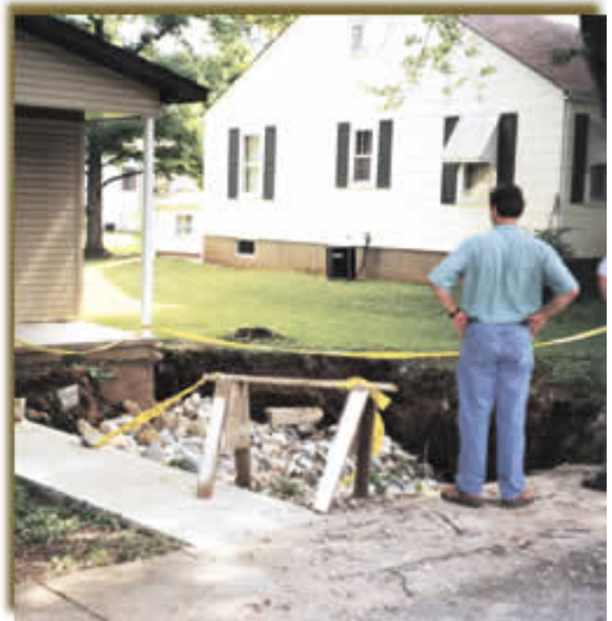
A sinkhole that formed in the front yard of a house in Farmington was partly repaired by placing large rocks in the bottom. DNR photo by Bill Dufey
