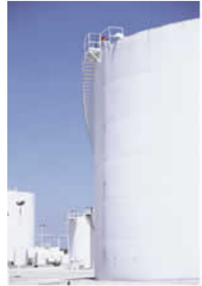
The "rack," at expansive terminals like Williams Pipeline near Columbia, sell gasoline at wholesale prices to local distributors. DNR photo by Scott Myers
