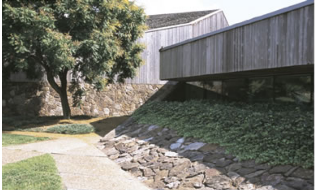
An insulating earthen berm and roof overhang that shades windows from summer sun are two of the design features that improve the energy efficiency of the Department of Natural Resources offices at 1659 E. Elm in Jefferson City. An upgrade of the building's heating, ventilation and air conditioning systems, light fixtures and office machinery, helped it earn designation as an Energy Star® building.
