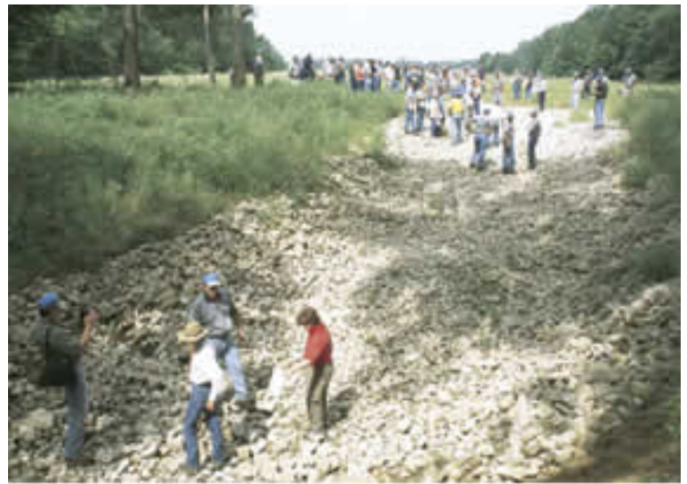
Field day participants examine a rock chute used to stabilize a stream bank and minimize erosion.
