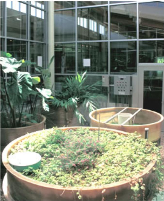
**The Living Machine uses a system of holding tanks and plants to clean wastewater that is generated at the Discovery Center. The water then is reused and routed to toilets inside the facility, as well as a wetlands outside.**
