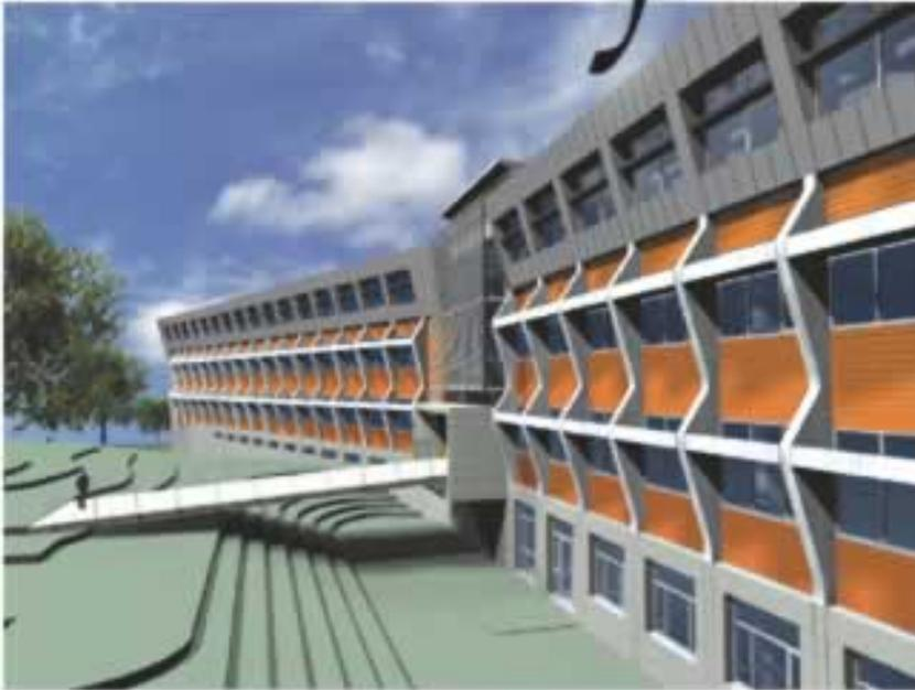
The exterior profile of the green office building helps capture and reflect light into the building significantly reducing the need for interior lighting.
