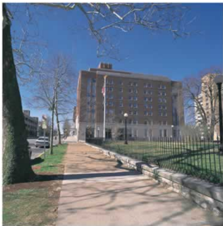
The late Gov. Mel Carnahan could see the deterioration occurring at the former Hotel Governor from the Governor's Mansion.
