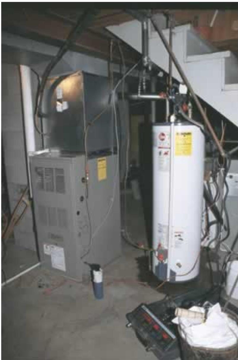
Diagnostic equipment tests the efficiency of a new hot water heater and furnace after the old appliances were replaced as part of the weatherization.
