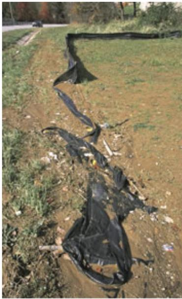
Collapsed fencing at a Columbia construction site contributes to erosion and sediment pollution.
