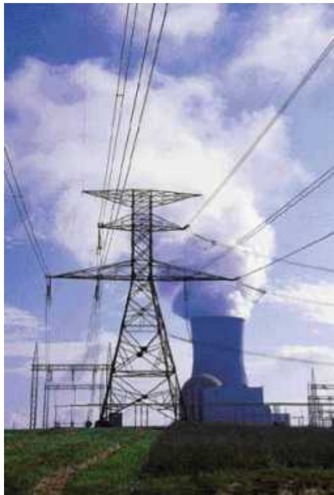
The enormous start-up costs of nuclear plants, like Callaway, might well give way to smaller, more numerous combined-combustion turbine facilities.
