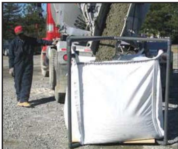
Figure 6.22 EnviroSac Concrete Washout Bag – Concrete Pump Supply, LLC.
