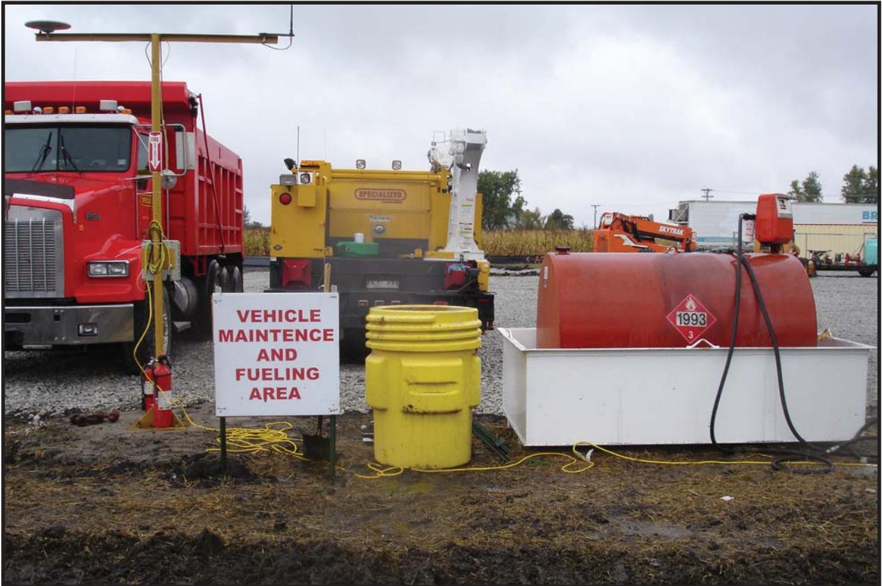
Figure 6.19 This site has a designated vehicle maintenance area with all petroleum products located within secondary containment areas. Source: BFA, Inc.
