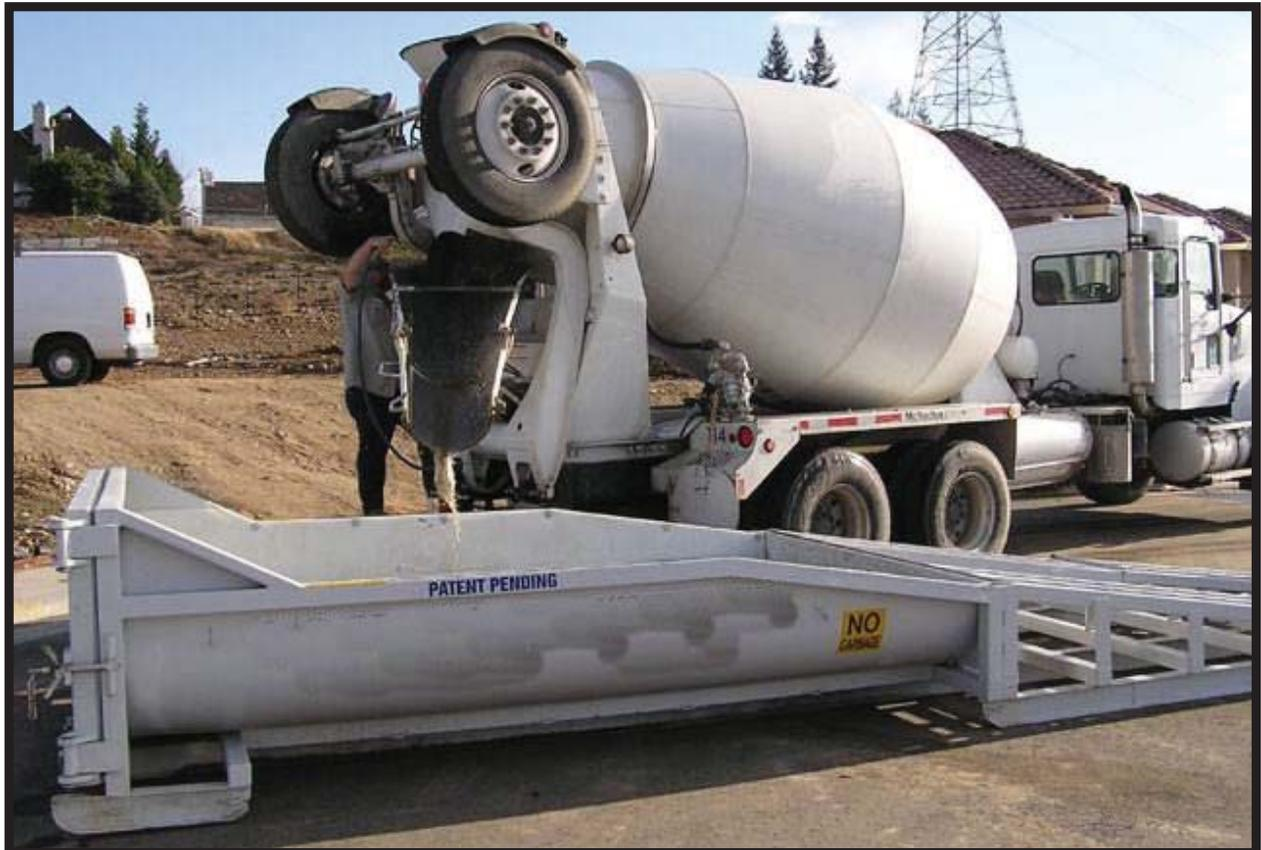
Figure 6.23 Concrete washout system that can be installed and maintained by vendor. Source: Concrete Washout Systems Inc.
