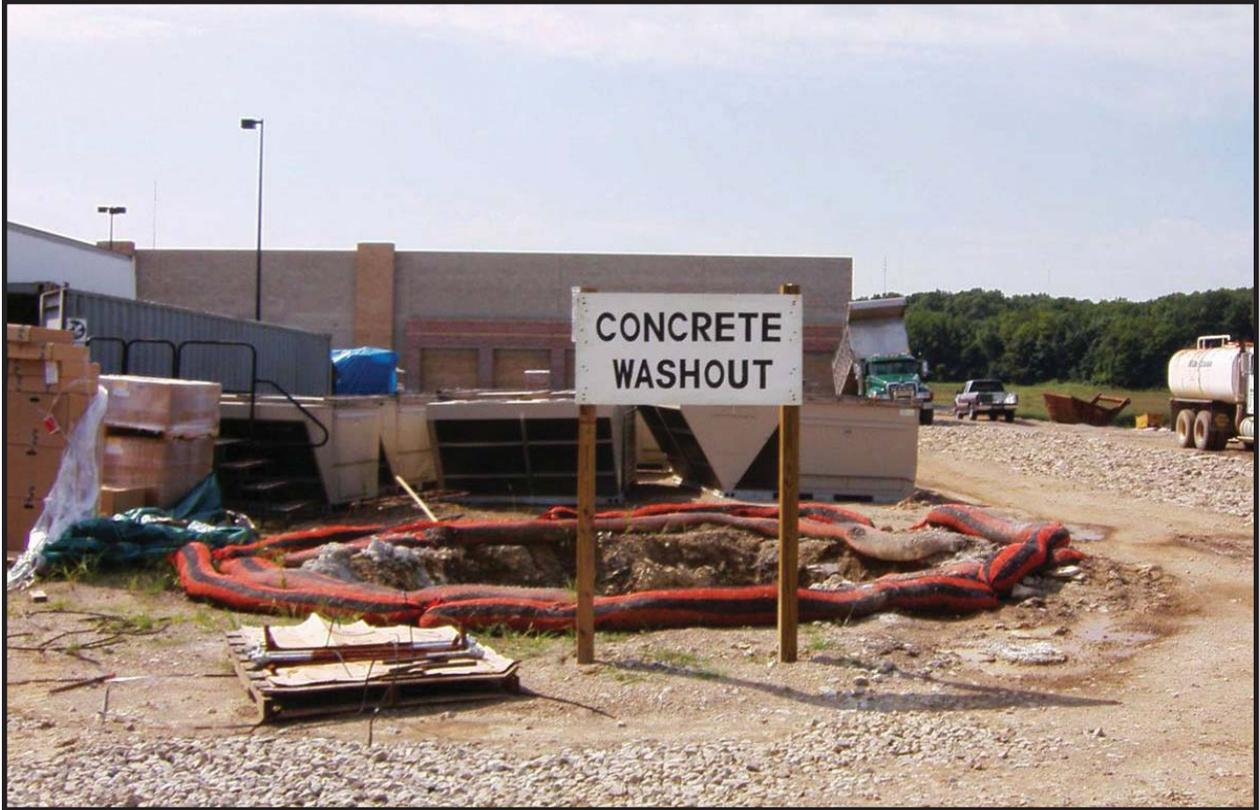
Figure 6.21 Concrete washout pit with signage. Source: ABC's of BMP's, LLC
