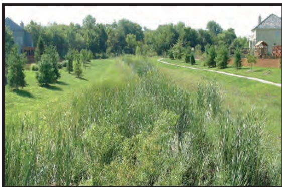
Figure 5.5 Wetland Swale. Source: Olsson Associates
