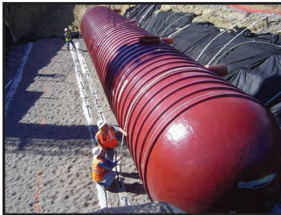
Installation of the water harvesting cisterns.
