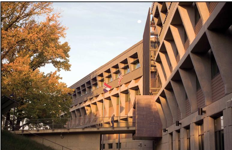
Large windows and light deflecting fins work together on the Lewis and Clark State Office Building to provide a brightly lit environment that does not heat up during the summer.
