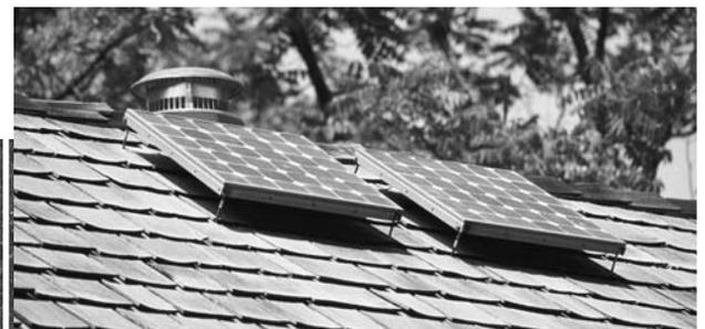
*In a remote location without electricity, this restroom at Ha Ha Tonka State Park uses photovoltaics to run exhaust fans. (Inset) The restroom’s roof-mounted solar panels are much more affordable than the cost of connecting an electrical line.*
