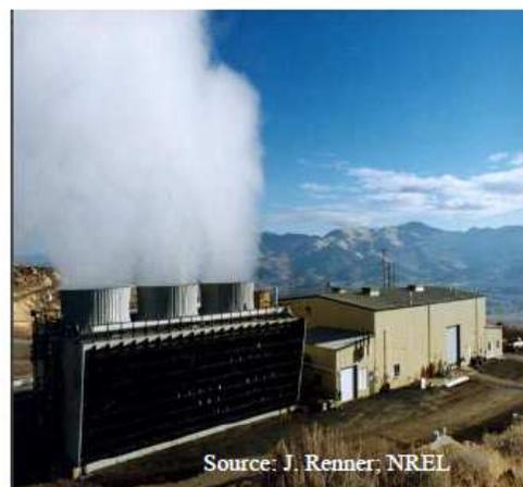
In some locations the available hydrothermal resources present more moderate temperatures. In these locations *binary cycle* systems can be used. A binary cycle plant passes the geothermal water through a loop called a heat exchanger and the thermal energy is transferred to a working fluid (usually isobutane) that boils at a low temperature. The vapor from the working fluid is then used to drive turbine systems and generate electrical power.
