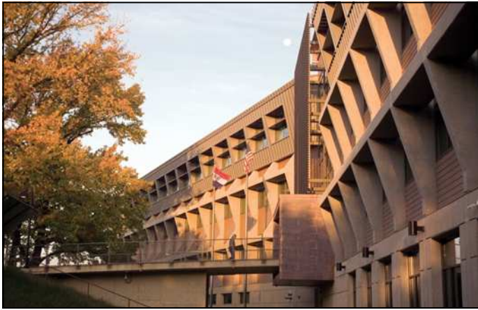
The Lewis and Clark State Office Building in Jefferson City utilizes passive solar design like these light shelves, among other methods, to increase energy efficiency.
