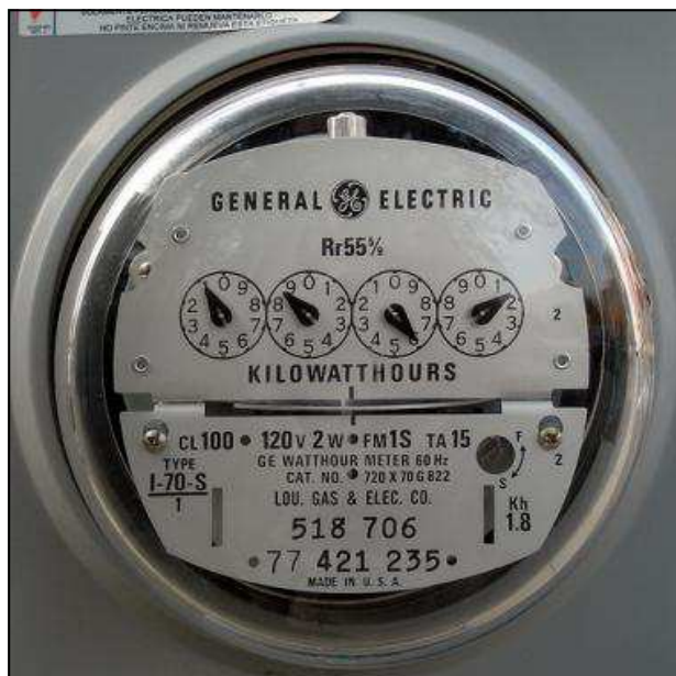
The standard electric meter tracks consumption for building owners and utility companies.
