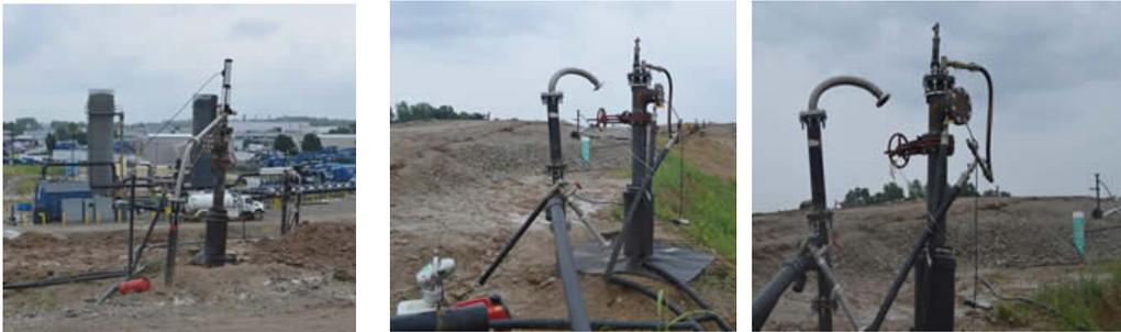
*Photos of Bridgeton Landfill's gas interceptor wells and TMPs.*
