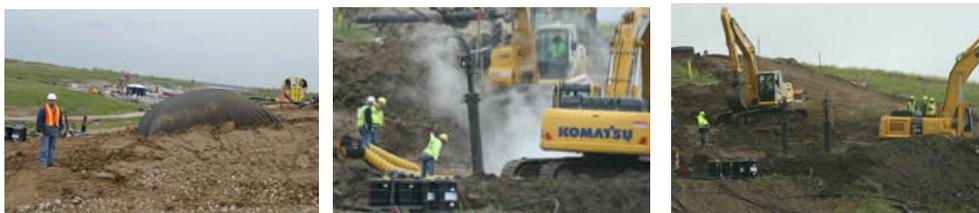
*Photos of SC-4 before abandonment with FML cover bulged and during construction activities in May, 2013.*
