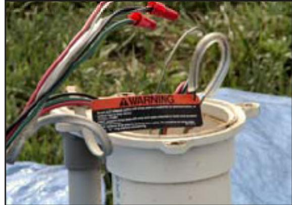
Wells with pitless units have the casing extending above the ground surface. Wells that have pitless adapter units have a cap over the well casing (sometimes they have three little set screws on the side of the cap to secure it).
