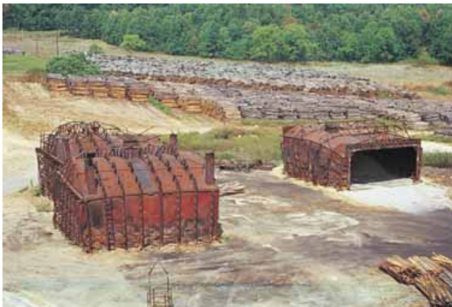
The old steel kilns at Royal Oak Enterprise's Mountain View plant now store finished charcoal.
