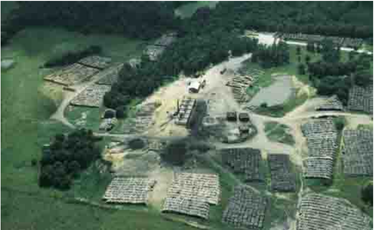
An aerial view shows six new emission-controlled charcoal kilns and the second-generation afterburner in operation near Mountain View. Preparations are under way for six more kilns and a second afterburner. DNR photo by Doug Elley
